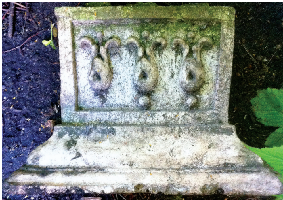
III. 2. Cast of detail of the townhouse at ul. Studencka 14 in Kraków made of hydraulic lime (photo by E.J. Sadowska)
