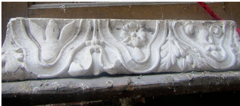
III. 3. Template used for recreating a fragment of the façade at ul. Studencka 14 in Kraków (photo by E.J. Sadowska)
