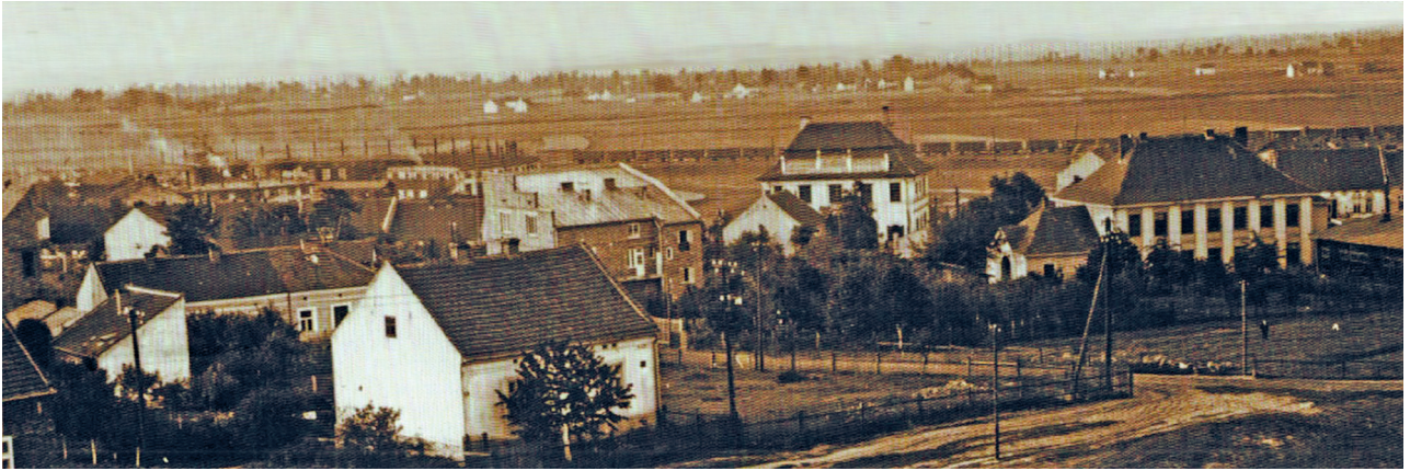
Fig. 2. The view on the railway settlement „Szutry” and meadow areas of Prokocim and Płaszów – 1930s.
