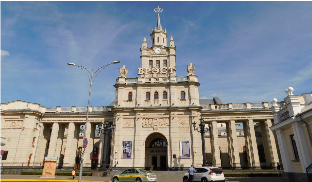
Fig. 4. Railway station Central Brest in 2019.
