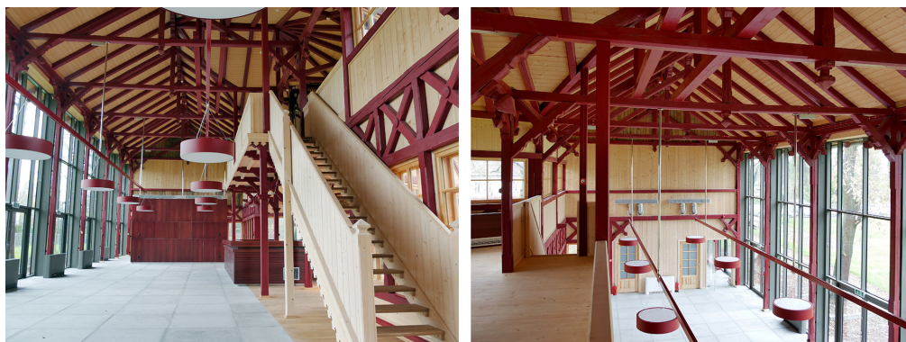
Fig. 10. View of the interior of the central segment. The open roof truss was restored by decorating it in the original colour scheme. The southern wall has been glazed to the entire height of the pavilion which was feasible after installation of a steel support structure (Source: Author's archive)
