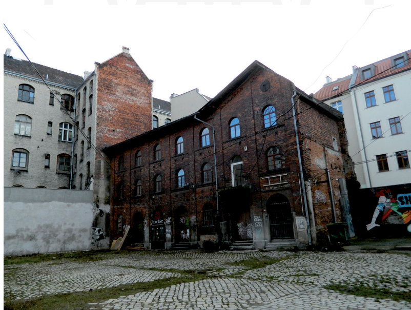
III. 6. Gable-end walls of houses in an unkempt backyard at Włodkowica Street show where no-longer-existing buildings used to stand. Original cobbles can be seen in the central part. Source: Chylińska (2013)
