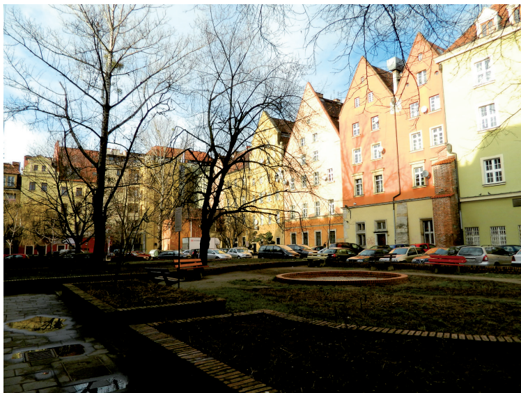
III. 3. Backyards situated behind the southern frontage of the Market Square in Wrocław are partly blocked with cars. Source: D. Chylińska (2013)
