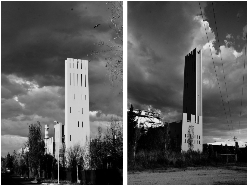
Fig. 3. Eco incineration plant – Riccone, near Rimini (photo by A. Wójtowicz-Wróbel, 2017)
