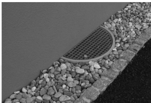
III. 3. Plinth of a new building with the rim of pebbles, Zurich, Switzerland
