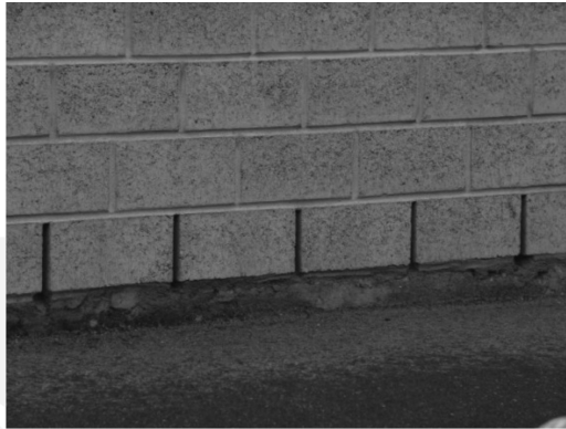
III. 9. Plinth of a new building with vent, Martini, Switzerland
