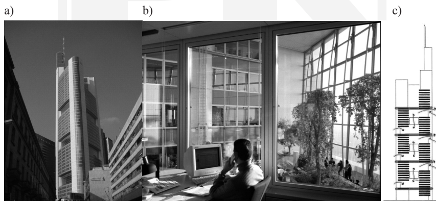
III. 4. Commerzbank Tower exterior facade, interior and ventilation scheme, Frankfurt am Main, Germany, 1997, design: Foster + Partners Ltd Riverside, 22 Hester Road London SW11 4AN (sources: a) author, b, c) [16])
