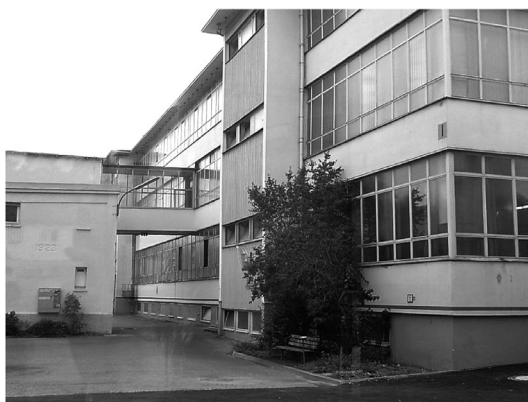
III. 2. Current state of the Steiff toy factory in Giengen, Germany (source: [13])
