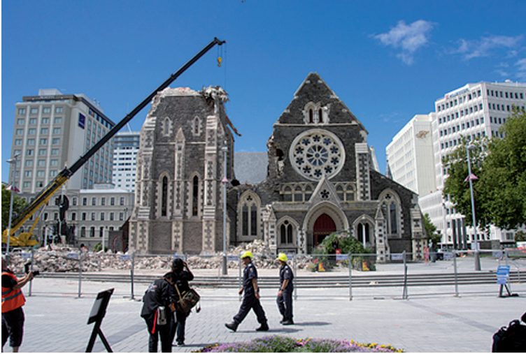
Illustration 1. Christchurch Cathedral after the February 2011 earthquake
