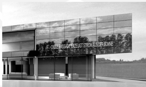
III. 4. Exposed facade with photovoltaics – Plus-energy-house, arch. P. Kuczia
