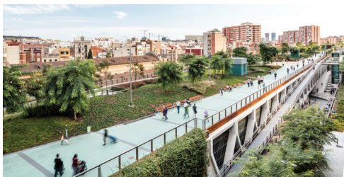
Fig. 22. Implementation of scenario S8: the JARDINES ELEVADOS DE SANTS project – surrounding structures and covering the railway line (a stretch of ca. 800 m, surface area of 48,400 m 2 ) with a city park in Rambla de Sants district in Barcelona, designed by Sergi Godia, A. Molino, arquitectos Esteyco Ingenieria ( https://www.plataformaarquitectura.cl/cl/801124/jardines-elevados-de-sants-en-barcelona-sergi-godia-plus-ana-molino-architects )
