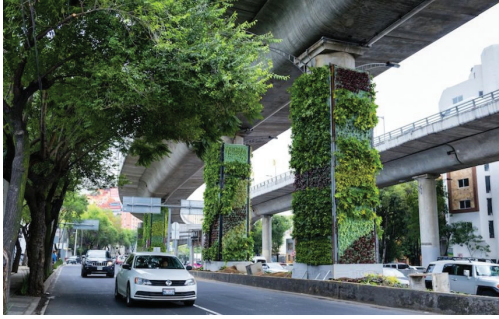
Fig. 24. Implementation of scenario S1: the VIA VERDE project – vertical gardens covering pillars of the flyover for Mexico City ring road (the gardens are intended to cover eventually 1000 pillars), designed by VerdMX ( https://www.thecivilengineer.org/news-center/latest-news/item/1157-vertical-gardens-in-mexico-city-to-combat-pollution )
