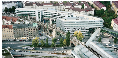
Fig. 23. Implementation of scenarios S9 and S10: design of an office and service building over a decommissioned flyover in Vienna (13,700 m 2 , length ca. 180 m), designed by Tillner und Willinger ZT GmbH, 2008 ( https://www.b2match.eu/system/building2017/files/01_TILLNER_ONLINEVERSION.pdf?1495443960 )
