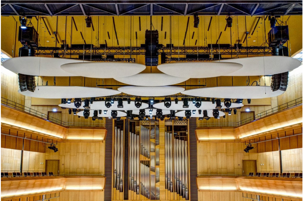
Fig. 4. Movable acoustic ceiling elements in Stavanger Concert Hall (source: [13])
