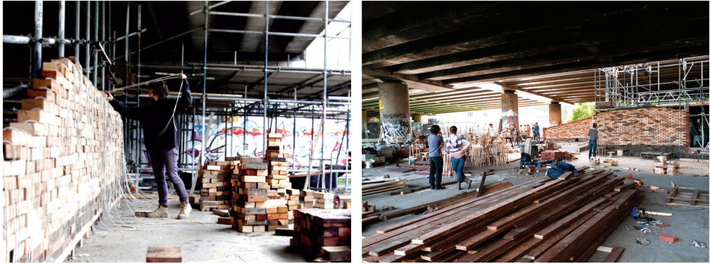
Fig. 5. Assemble, Folly for a Flyover (work in progress), photo by Assemble [8]
