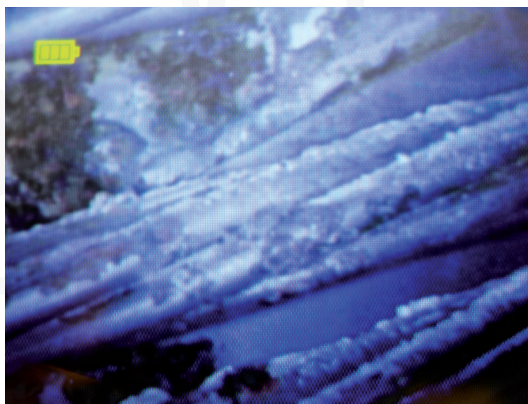
Fig. 6. View of the interior of the prestressing cable duct
