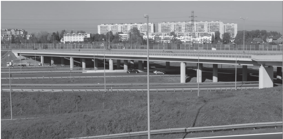
Fig. 1. View of the structure
