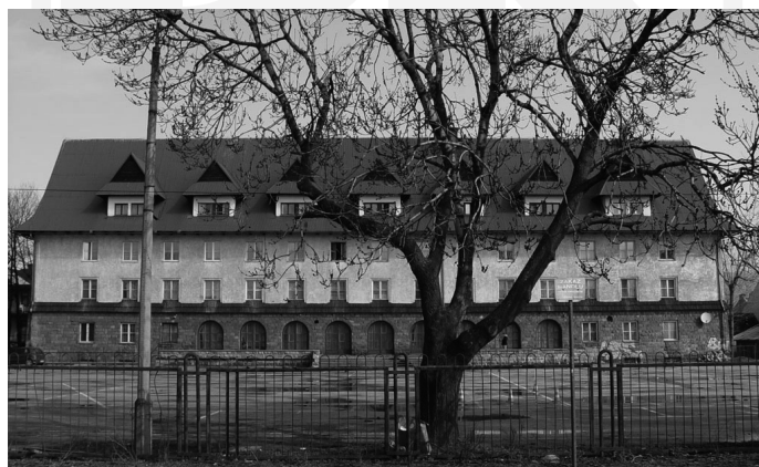
Ill. 2. View of the dormitory building in Nowy Targ from the south (from Al. Tysiąclecia) before project intervention, November 2008 (photo: D. Kuśnierz-Krupa)
