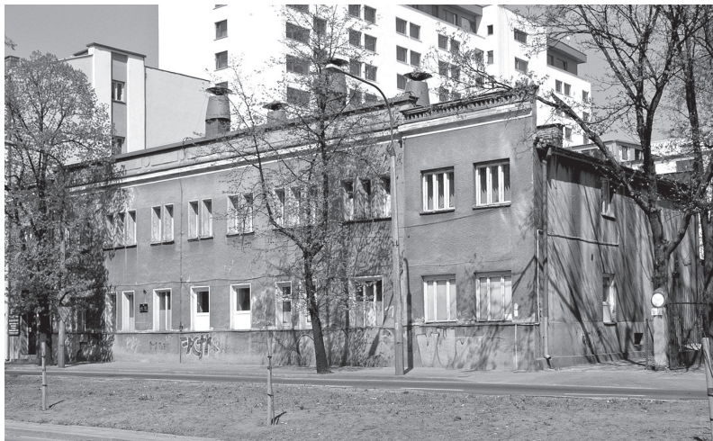
Fig. 7. The Samuel Mohilewer synagogue – adaptation and extension, 2013 (photo by Piotr Trojnieł)
