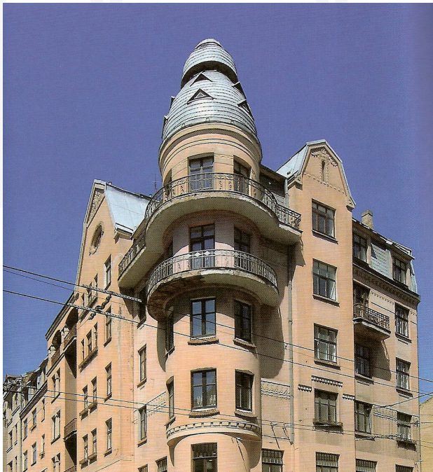
Fig. 27. Multifunctional building. Riga. A. Vanags, 1911
