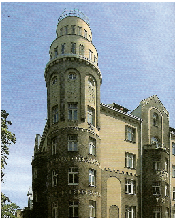
Fig. 29. Multifunctional building. Riga. R.P. Dohnberg 1910
