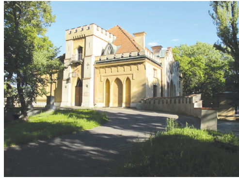
Fig. 4. Residential complex Mokotów, Warsaw (photo by K. Pluta, 2016)
