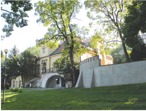
Fig. 3. Residential complex Mokotów, Warsaw (photo by K. Pluta, 2016)
