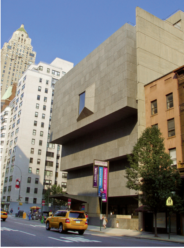
Ill. 8. The western façade makes part of the Madison Avenue frontage (photo by W. Gadomska)
