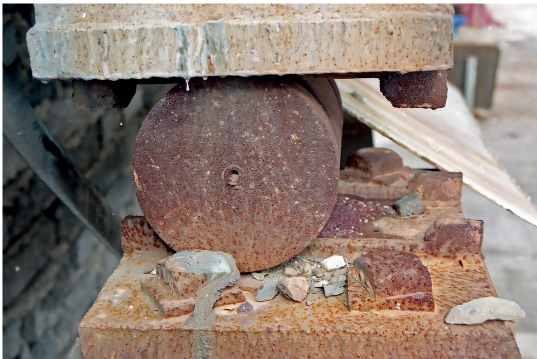
Fig. 5. Eastern lower bearing
