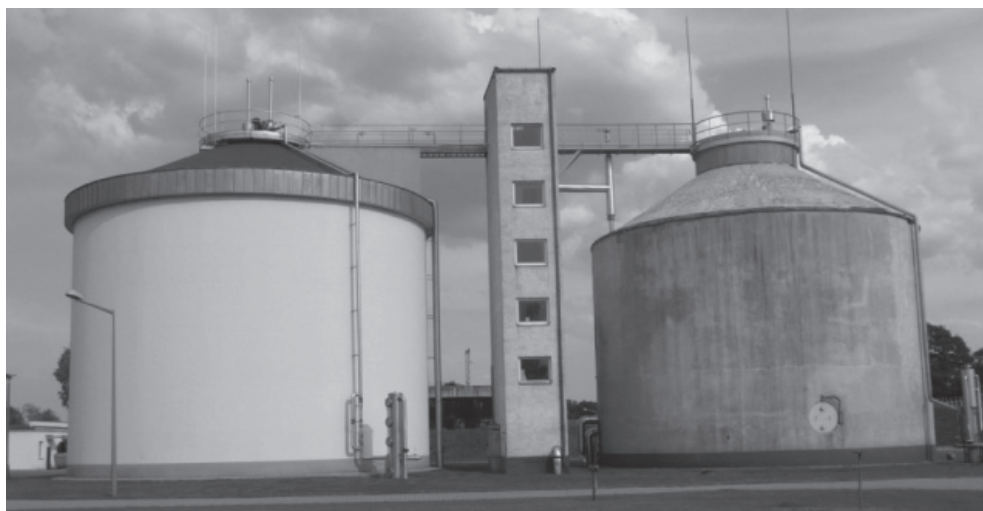
Fig. 1. The view of the two digestion chamber tanks (analysed tank on the right)
