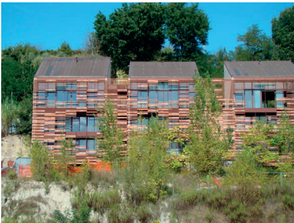
III. 7. Colle Fabbričina. New residential development, proj. by Jean Nouvel (photo by author, 09.2014)
