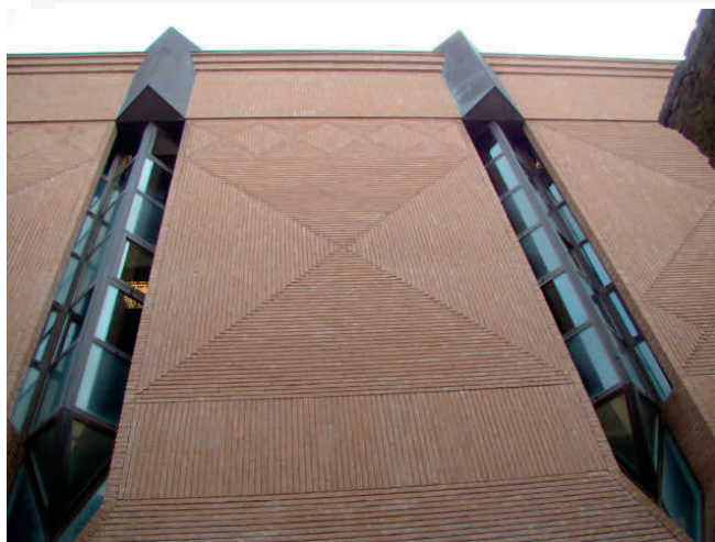
III. 3, 4. Volterra. New Town Museum in the structure of a mediaeval city (photo by author, 09.2014)
