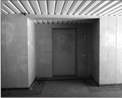
Fot. 1. Zamurowany szyb windy na dworcu Łódź Kaliska (fot. P. Kosmowski) Photo 1. Bricked-up elevator at the station Łódź Kaliska (photo by P. Kosmowski)
