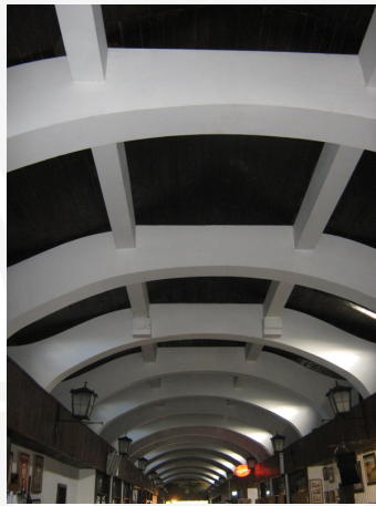
Fig. 9. The ceiling beams in the reconstructed bridge in Lovech (photo by D. Partov, 2013)
