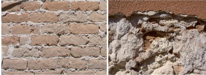
III. 8. Photos present the deterioration of the masonry structure of the external walls
