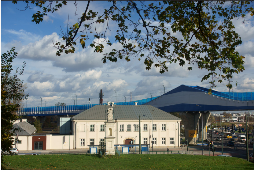
Illustration 3 Museum of Podgórze in Krakow located in the St. Benedict Inn. Behind the building the railway flyover. Photo Paweł Kubisztal
