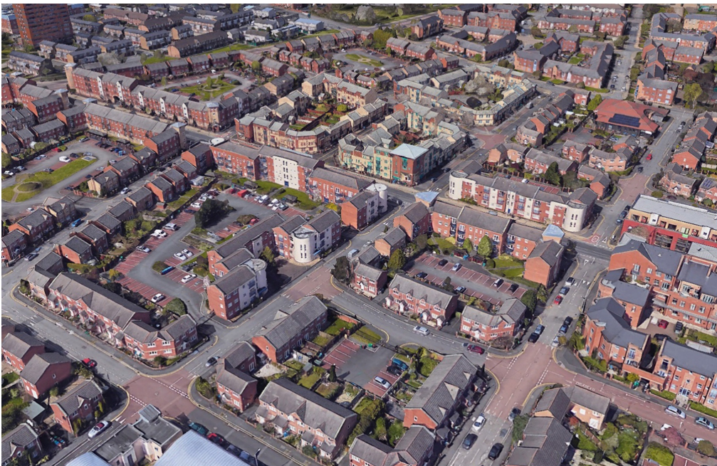
Fig. 15. Development quarters in the central part of the district (source: [25])
