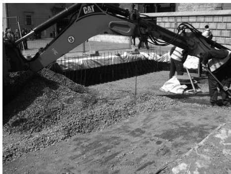
Fig. 3. Methods of strengthening weak soil: a) in the lower left corner the originally designed strengthening using geogrid can be seen, b) The said geocell (source: Royal Castle on Wawel Hill archives)
