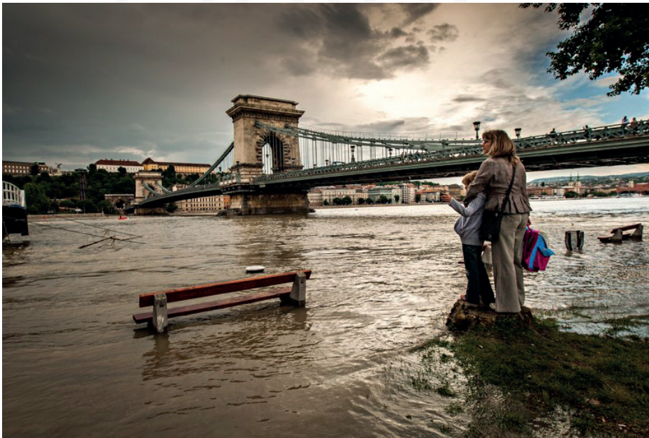
Fig. 1. The summer flood 2013 of Danube River caused costs of over ten Mio. Euro for Budapest, Hungary [4]. At 17th of August 2013 96 mm of rain fall within one hour– an amount equivalent to the average of one month. Consequently, the canal system could not cope with the runoff and on some streets flow more than one meter high water.[5]
