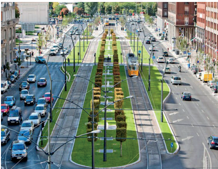
Fig. 6. Rehabilitation of Károly-körút [21]
