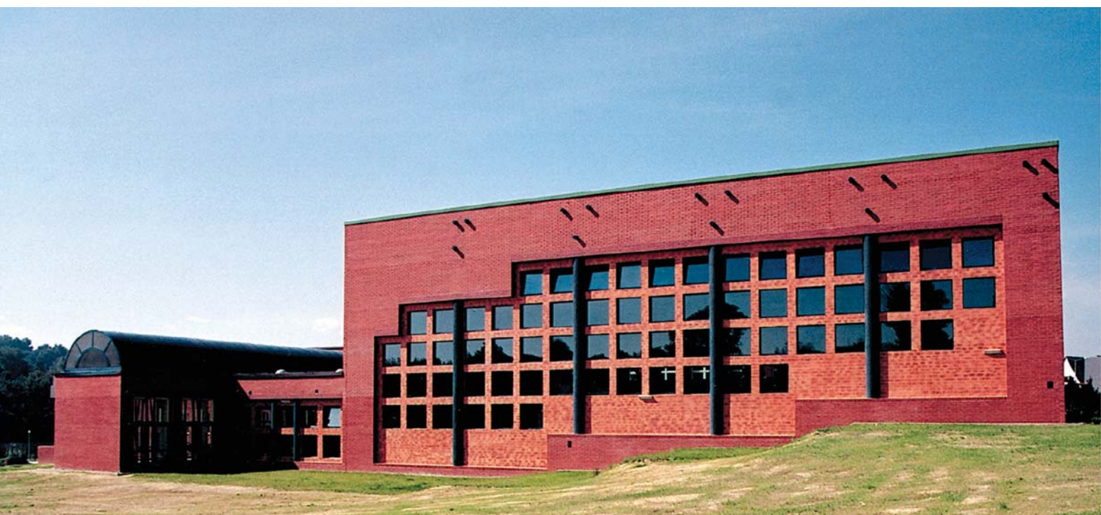
III. 10,11. Junior high school with a sports hall within the scheme of a school complex. Skawina, 3 Witosa street 1997-2001. Authors: Wacław Seruga main designer, Małgorzata Buratyńska-Seruga, Kazimierz Hamada. 1st Award – Competition of the Union of Polish Architects Branch in Cracow 1994, Grand Prix – Competition "Miss of Clinker" 2002, Distinction of the Polish Union of Civil Engineers and Technicians – All-Poland's Competition "Construction of the Year 2001". Photo: Wacław Seruga
