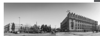
1. Buildings of the Administrative Centre of the Lenin Steelworks. Photo by Igor Stanisławski → see p. 164
