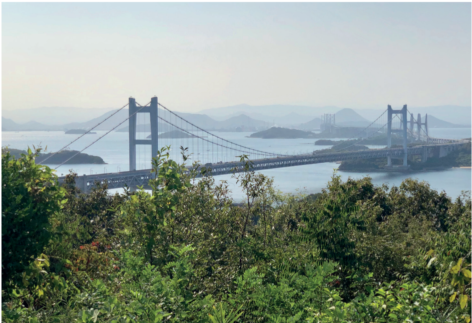
7d. Shimotsui Seto Ōhashi Bridge
