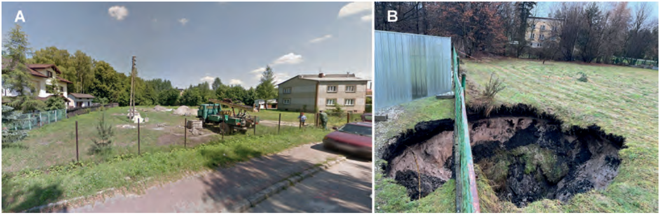
Fig. 10. A) Injection of filling material to the loose zones in 2013 ( www.google.com/maps – street view); B) the sinkhole appearing in the survey site in December 2022 ( https://wiadomosci.onet.pl/krakow/ ) – detail location is shown in Fig. 2C
