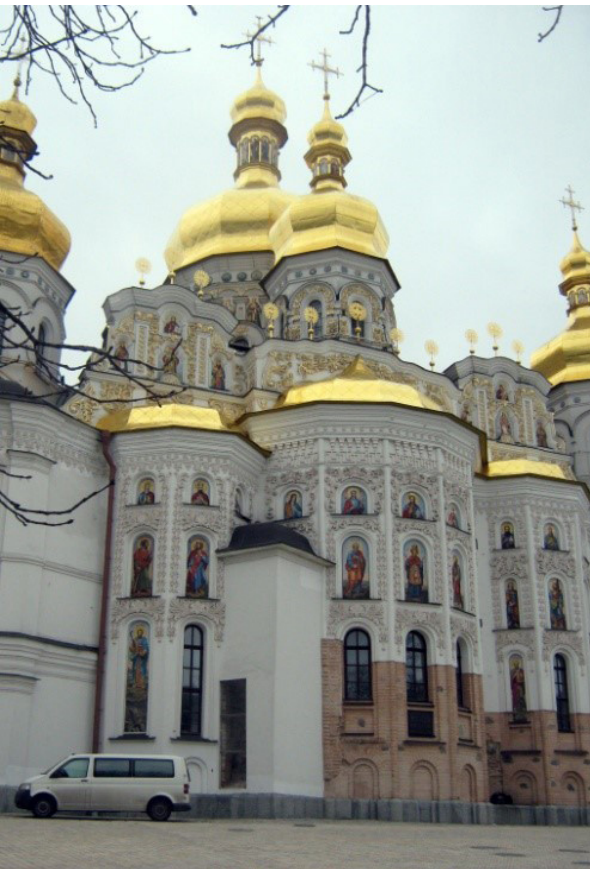
Ill. 4. Preserved original ruins which were integrated into the new structure of The Assumption Cathedral of Kyiv-Pechersk Lavra. Photo by S.Linda, 2020
