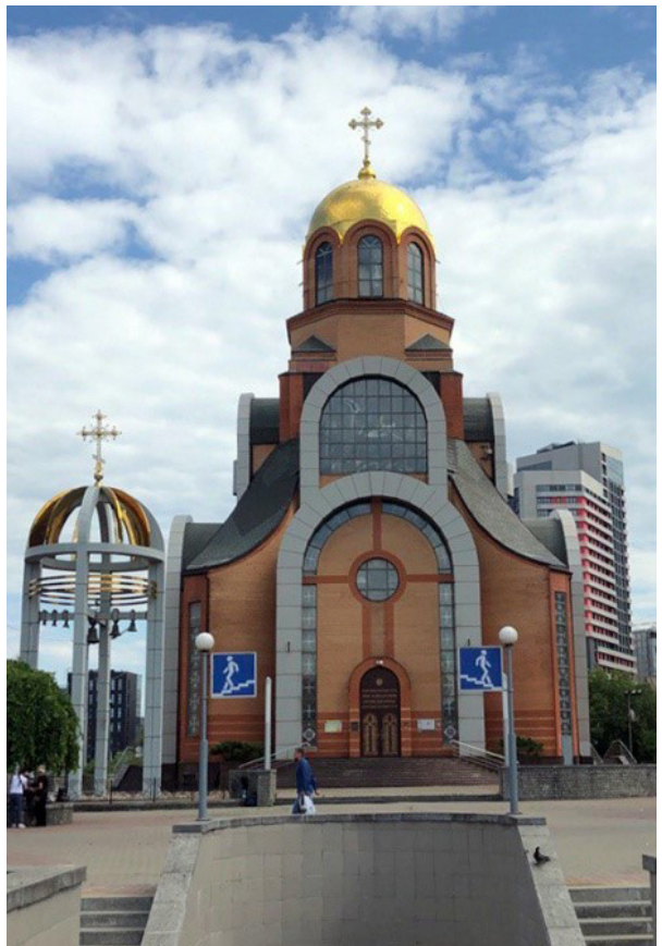
III. 7. The Church of St. George the Victorious for the workers of the Ukrainian Railway in Kyiv, 1998-2001, arch. R. Syvenkyi. Photo by S.Linda, 2022
