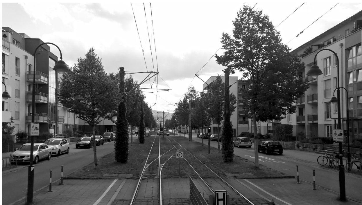
III. 4. Freiburg i.Br. - perspective view of Rieselfeldallee. A typical green alignment in central reservation between single-lane carriageways; photo: Jacek Wesołowski, 2015
