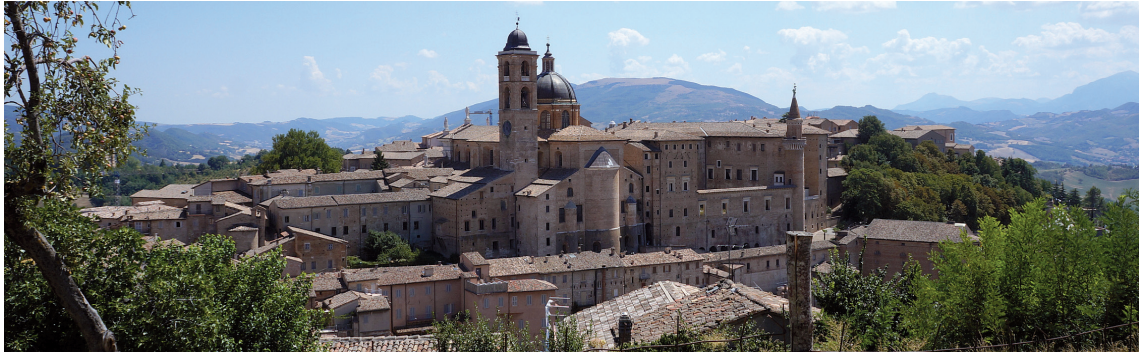
III. 14. Urbino – homogeneity implemented in a different material (brick) characteristic of the region of Marche
