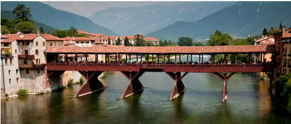
Fig. 10. The current state of a wooden covered bridge Ponte degli Alpini in Bassano del Grappa (source: https://anotherheader.wordpress.com/2010/12/23/italy-bassano-del-grappa , access: April, 2016)
