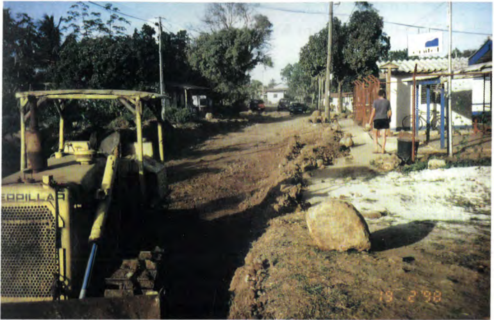
9. New „Enitel” telephone company and roadworks
