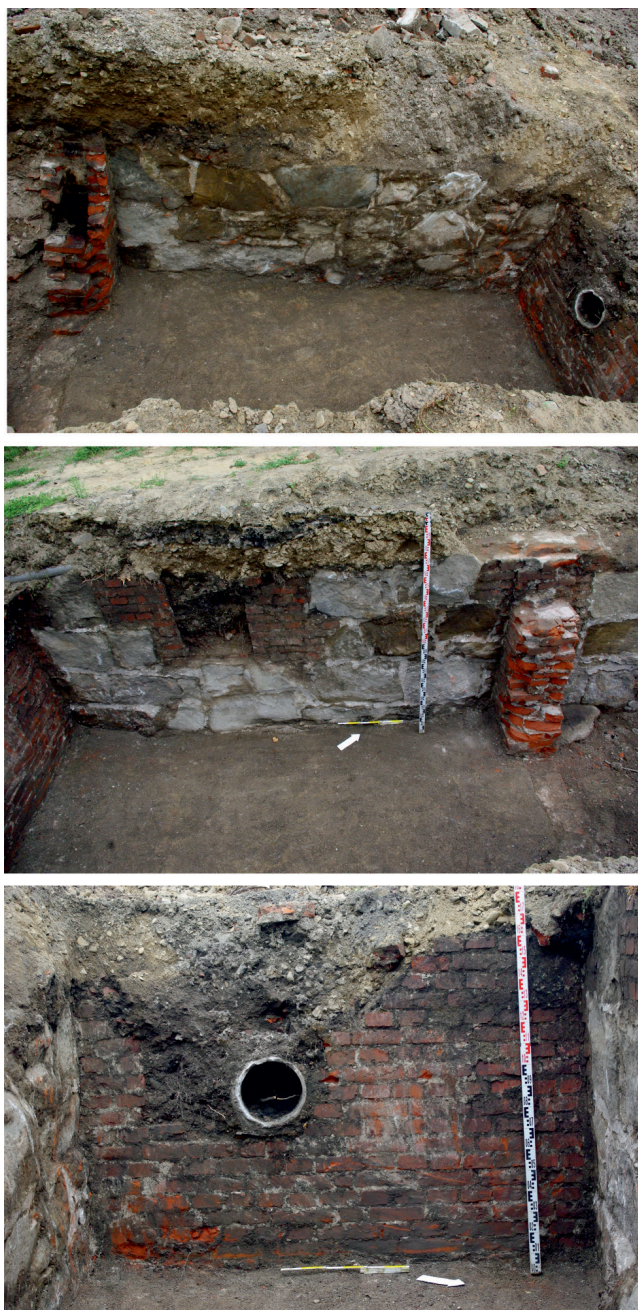
FIG. 14. Relicts of walls and rooms of Police Station from end of 19 th century (photo P. Kocańda)
