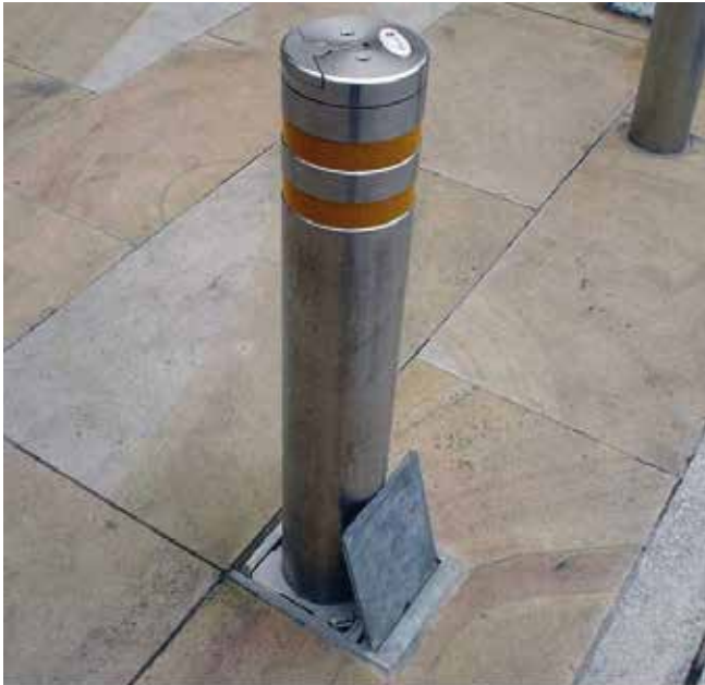
Image 8. Manually controlled bollard.
