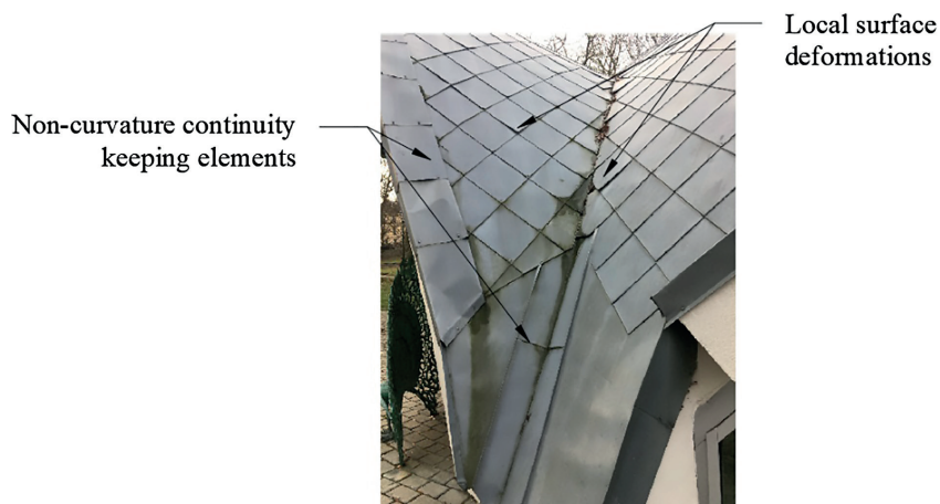
Fig. 4. Local surface deformations and elements not keeping curvature continuity
