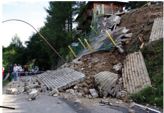
Fig. 2. Landslide on national road No. 87, 28 June 2009 [26]
