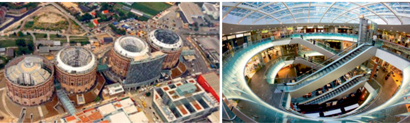
ill. 3. General view and interior of the shopping and entertainment center «Gasometer City» in Vienna, https://twistedstifter.com/2009/10/gasometers-of-vienna/
