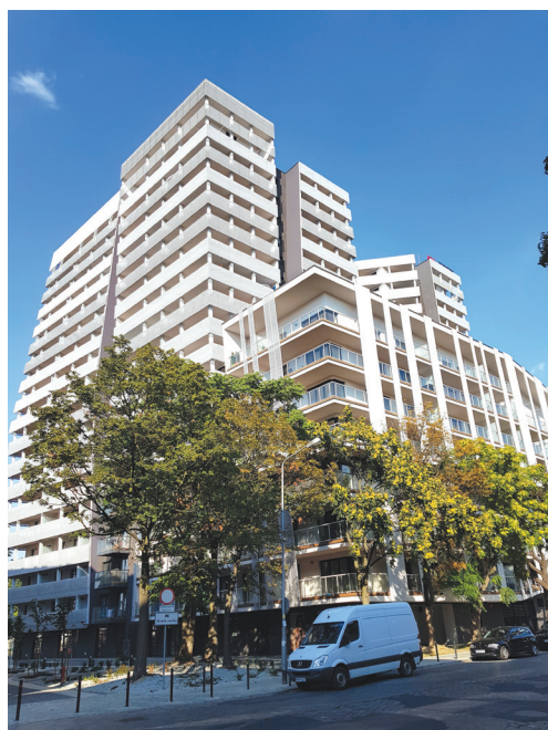
Fig. 2. ATAL Towers – Part II – eighteen-storey towers with a lower, eight-storey base, view towards the east from Generała Sikorskiego Street
