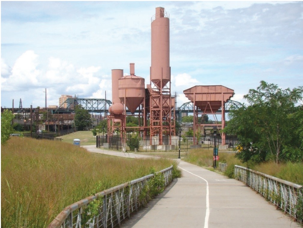
Fig. 10. Technical infrastructure exposed in the park space (photo by W. Gadomska)
