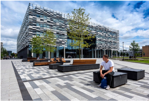
Fig. 20. Brook Building (source: [28])
