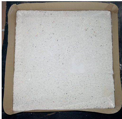
Fig. 4. Concrete substrate after the grinding process
