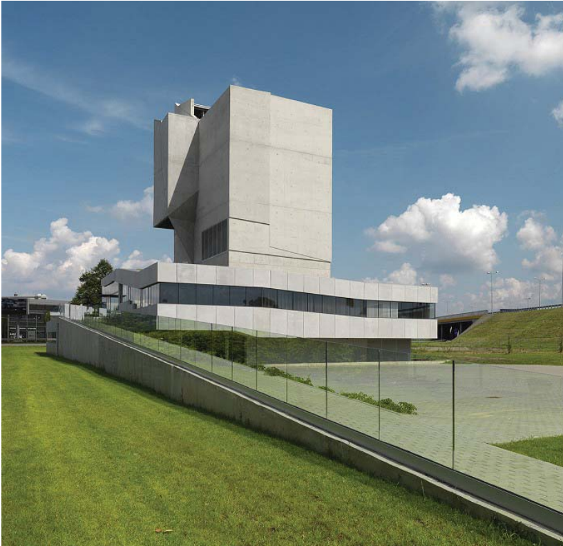
Fig. 4. Lewicki and Latak Studio, Aerotunnel in Mory, 2014
