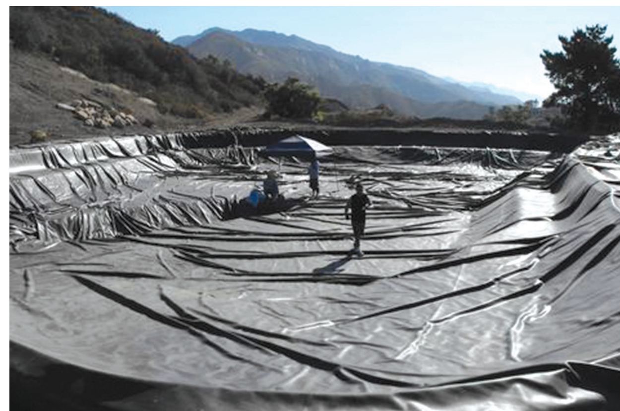
ill. 6. Organization of an artificial lake using polymeric materials in the natural landscape; https://justpondliners.com/collections/commercial-use
