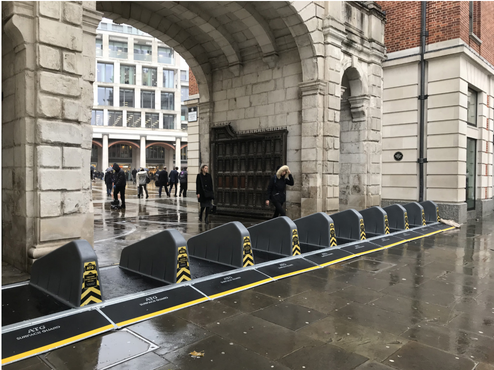
Fig. 4. “Surface Guard” temporary barrier in a city centre street (source: [1])
