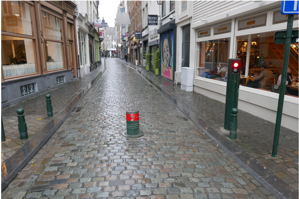
Fig. 7. Remotely-controlled hydraulic bollards blocking access to an inner-city pedestrian zone in Brussels (photo by A. Jasiński)
