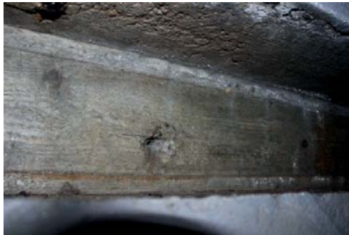
Fig. 8. View of left fragment of wooden formwork (own photo)
