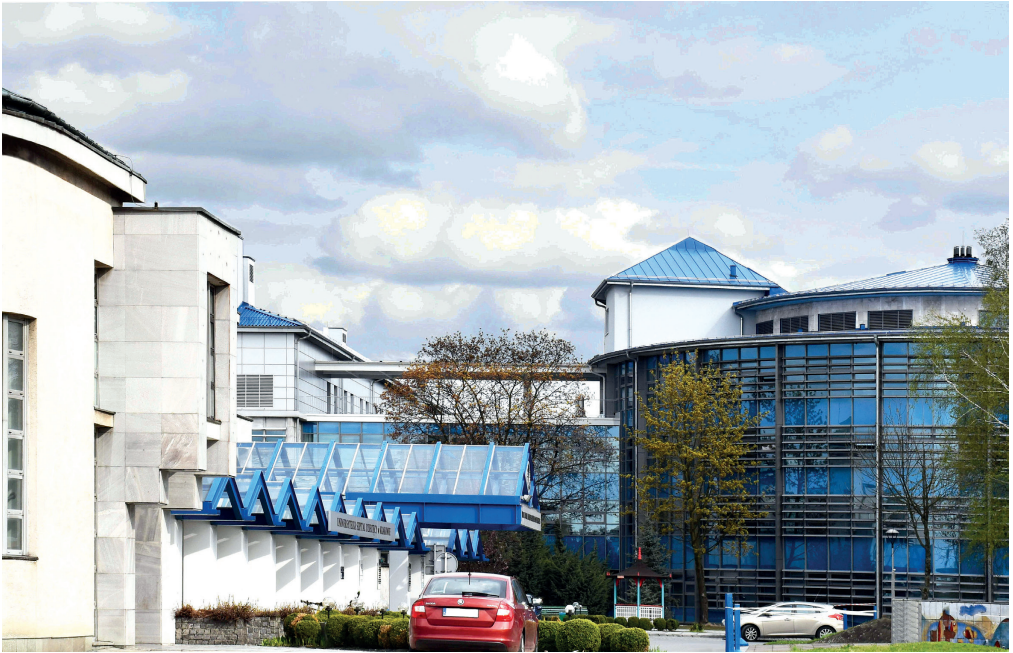
Fig. 3. The Children's University Hospital in Cracow, view of the Children's Outpatient Treatment Centre (CALD) from beginning of 90. and the oldest part of the hospital after renovation and modernization (photo by E. Waszczyszyn, 20.04.2017)
