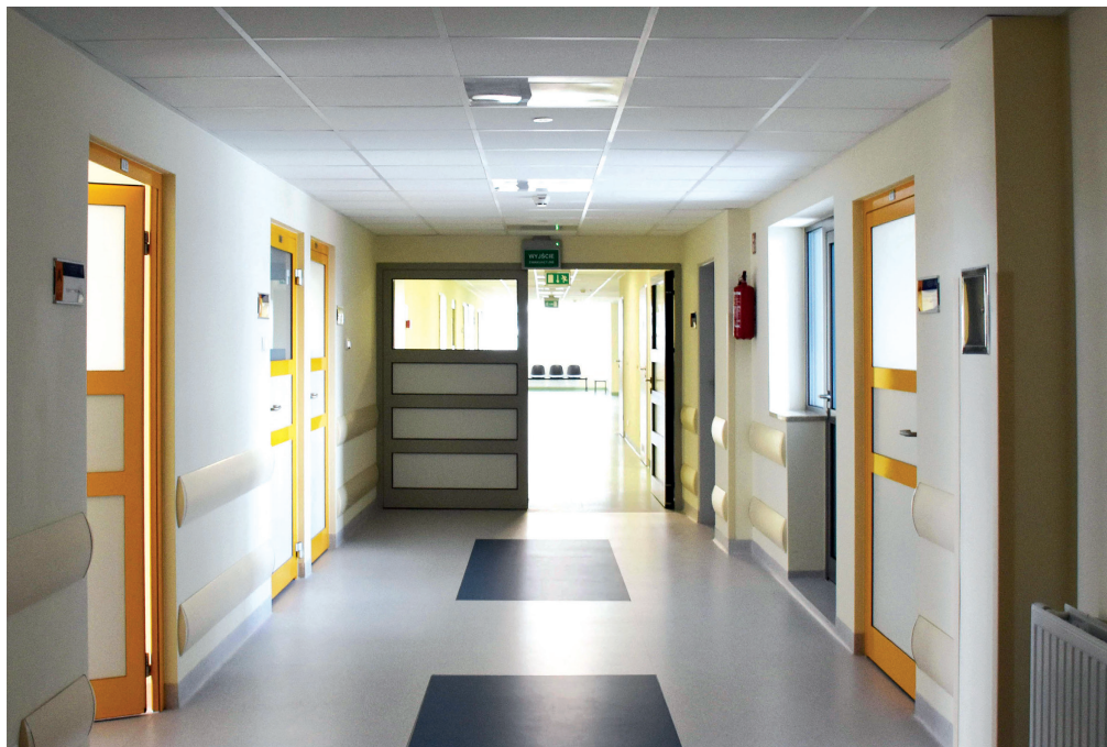
Fig. 9. Children's University Hospital in Cracow, view of the interior of the oldest part of the hospital after renovation and modernization, hospital corridor (photo by E. Waszczyszyn, 20.04.2017)
