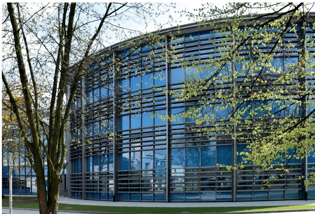
Fig. 5. Children's University Hospital in Cracow, view of the oldest part of the hospital after renovation and modernization (photo by E. Waszczyszyn, 20.04.2017)
