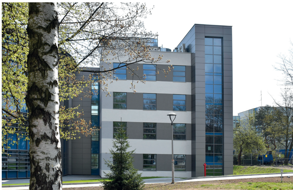
Fig. 8. Children's University Hospital in Cracow, view of the expanded part of the oldest part of the hospital after renovation and modernization (photo by E. Waszczyszyn, 20.04.2017)
